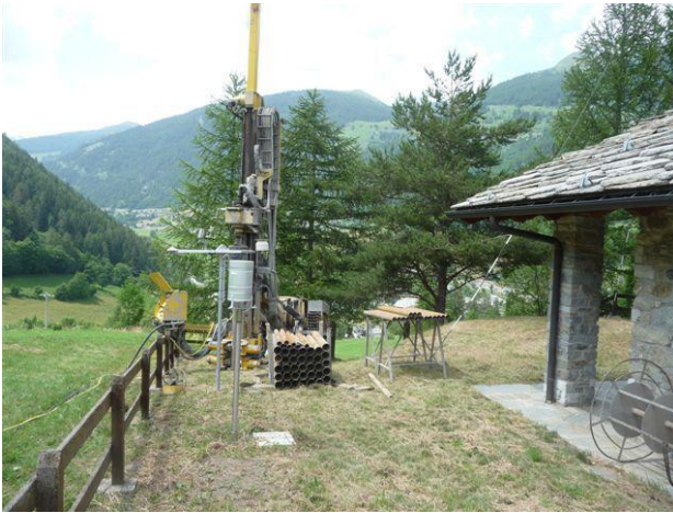
Fig. 3. View of the pilot site during drilling phase.
