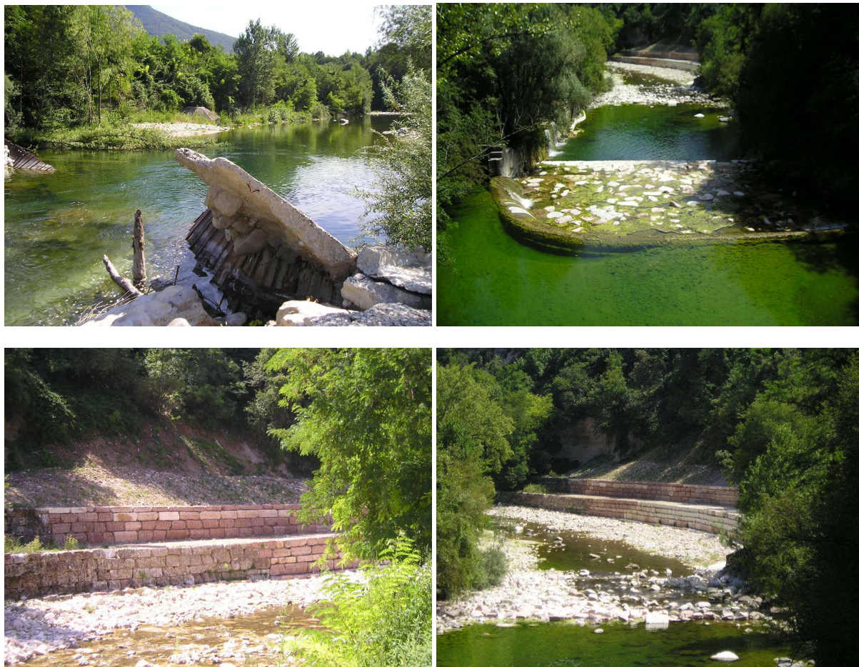
Figure 28: transversal and longitudinal hydraulic works along the Astico analyzed river reach
