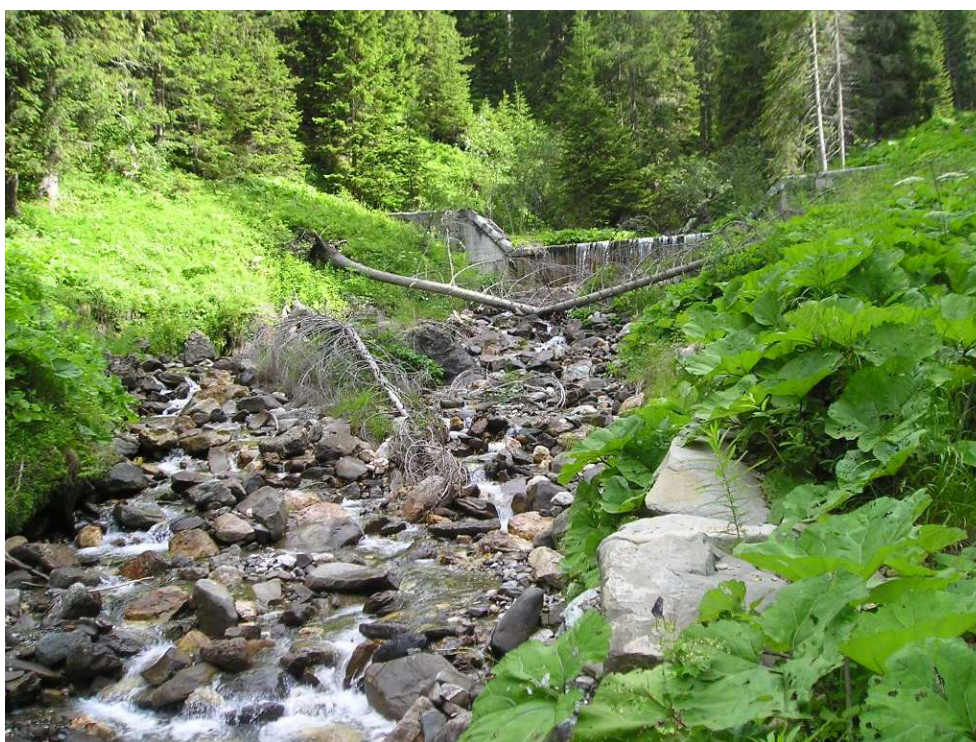
Figure 77: check dams along the channel reach downstream the withdrawal point
