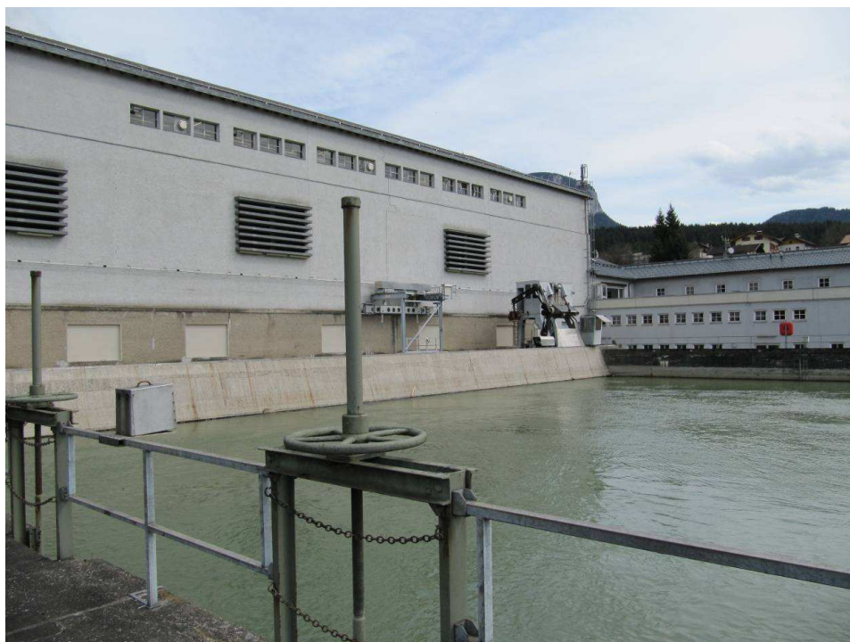
Figure 17: The power house of the HP Kirchbichl.
