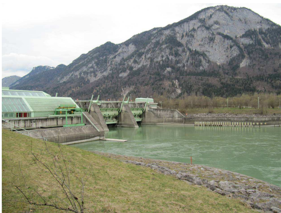
Figure 18: The power house and the weir of the HP Langkampfen seen from the downstream side.
