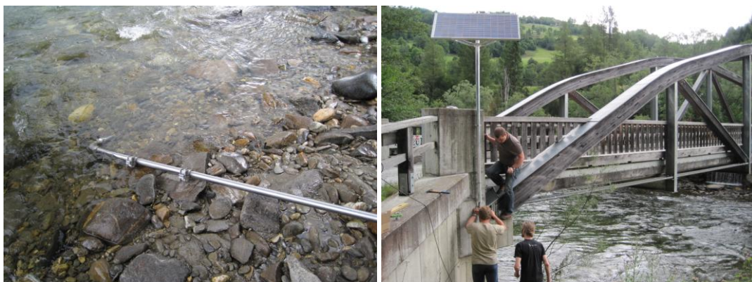
Figure 7: Installation of the turbidity probe at Wandritsch bridge
