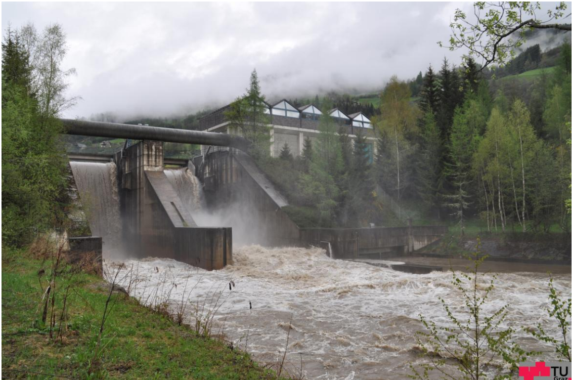
Figure 1: Hydro power plant Bodendorf during flood
