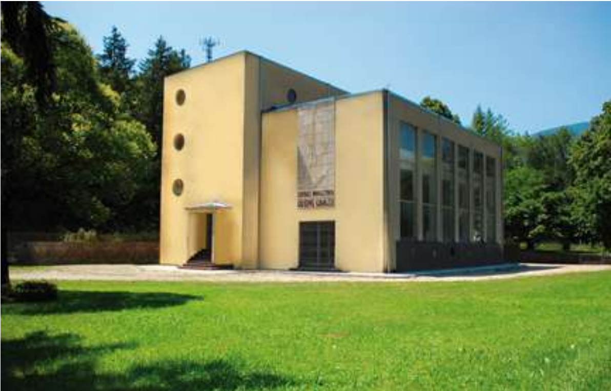
Bessé's hydropower plant
