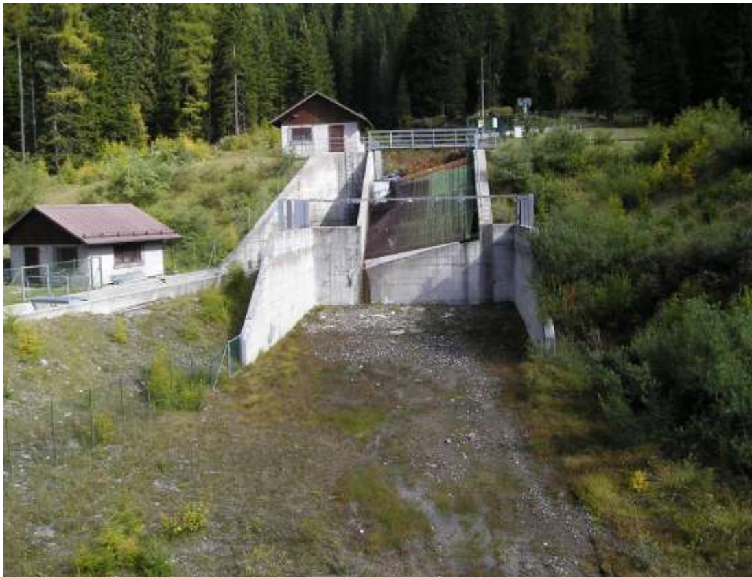
ARPAV's solid discharge measuring station
