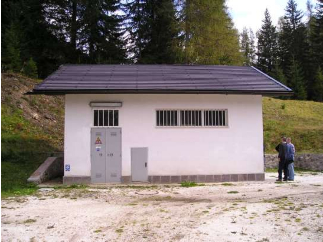
BIM HP plant located at 1468 m a.s.l.
