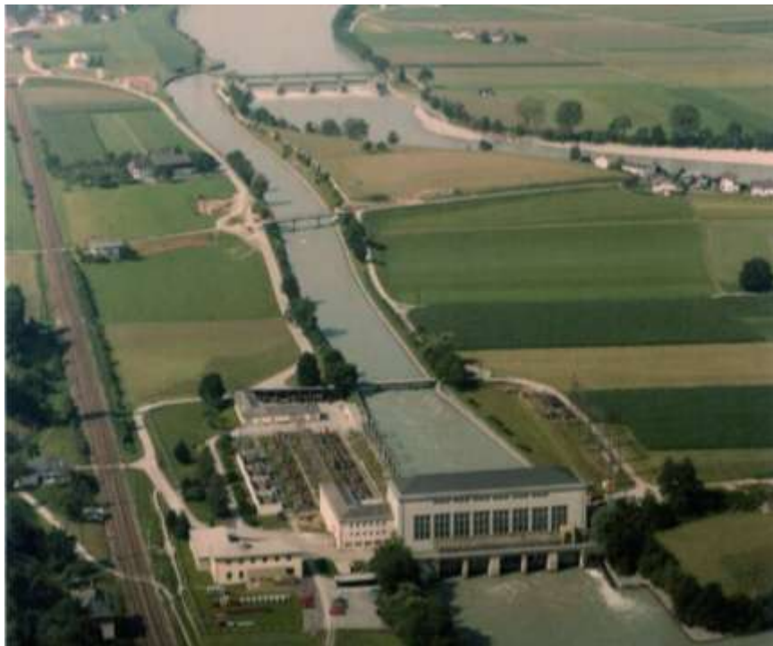
Image 1: Powerhouse, water channel, residul-water and weir of the hydropower-plant Kirchbichl in the river Inn (Picture: TIWAG).
