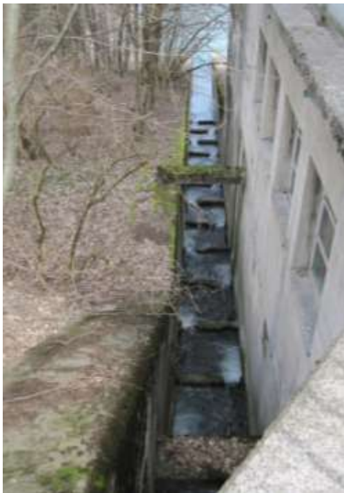
Image 13: Fish ladder (Picture: Baldes)
