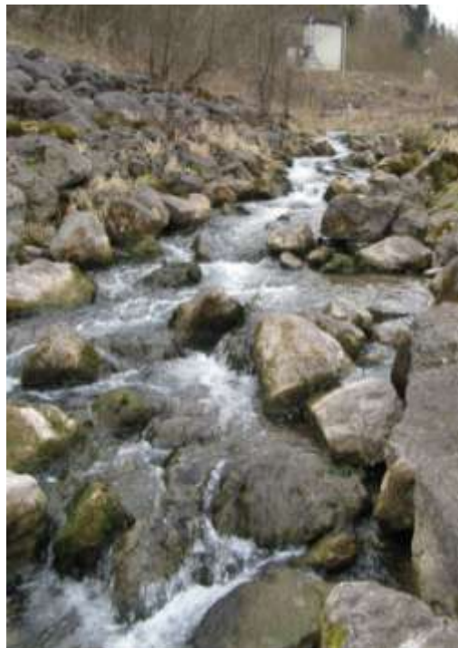
Image 14: Fish bypass (Picture: Baldes)
