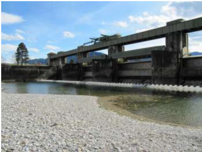
Image 2: The weir at the upper side of the meander (picture: Baldes)
